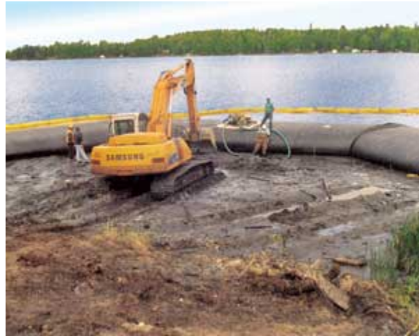
Sediment removal behind coffer dam
